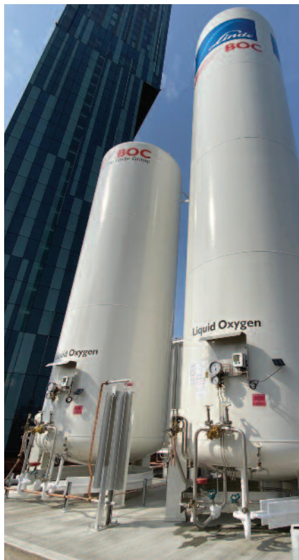
It was agreed that the site needed at least one vacuum insulated evaporator (VIE) unit.
